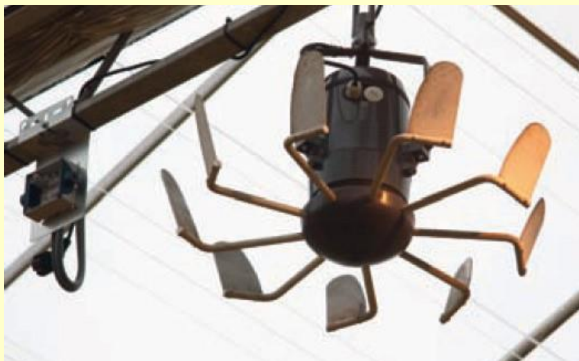
The special design of the vanes results in the displacement of air masses from the bottom to the top, and vice versa.
