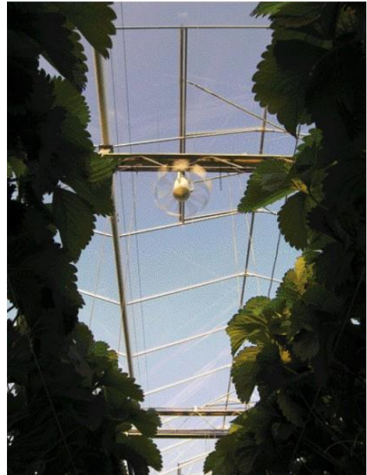
One Aircobreeze fan per 200 square metres creates an air current of 5 centimetres per second – with a low power consumption of 1 Watt per square metre.
